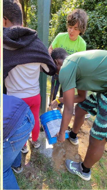
Pouring concrete after getting the kiosk into position
