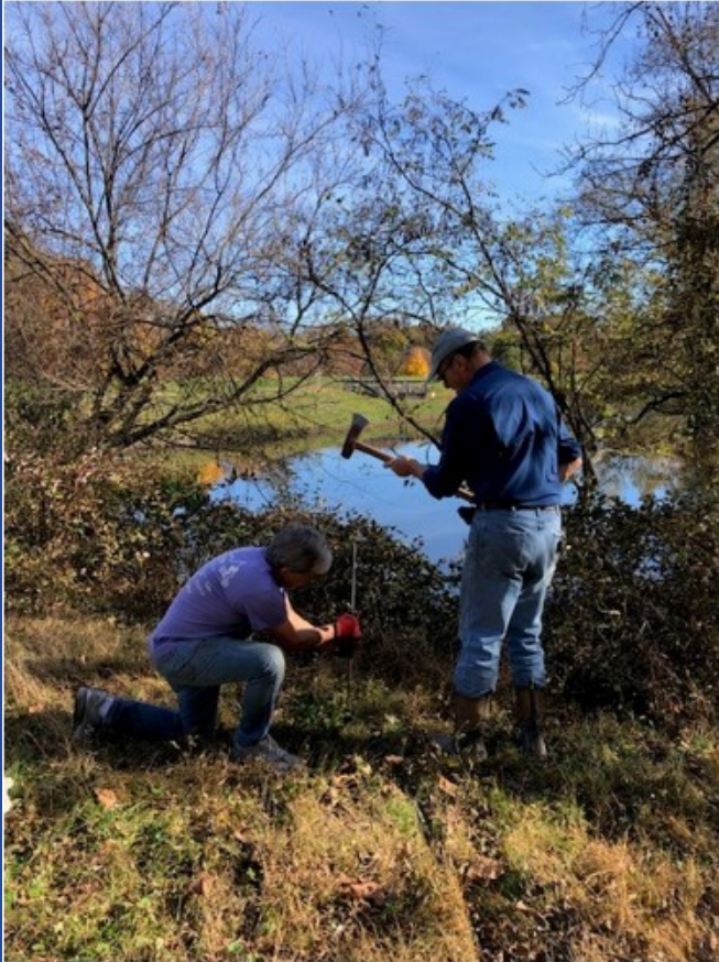
Walter Mulbry (at left) and Ken Klein installing the base of a nest box
