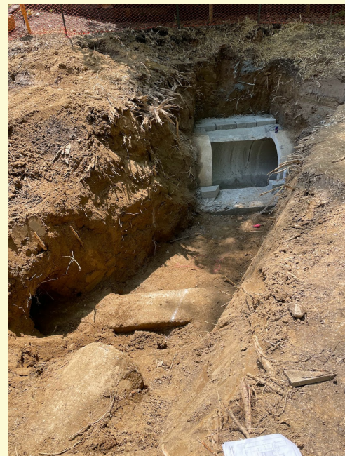
The restored storm drain pipe (at right) carries overflow into the storm drain system, which drains into Sligo Creek. Perforated piping (at left) in the bioretention media, roughly 2.5 feet below the surface, helps distribute the water throughout the bioretention area. (MCDOT photos)
