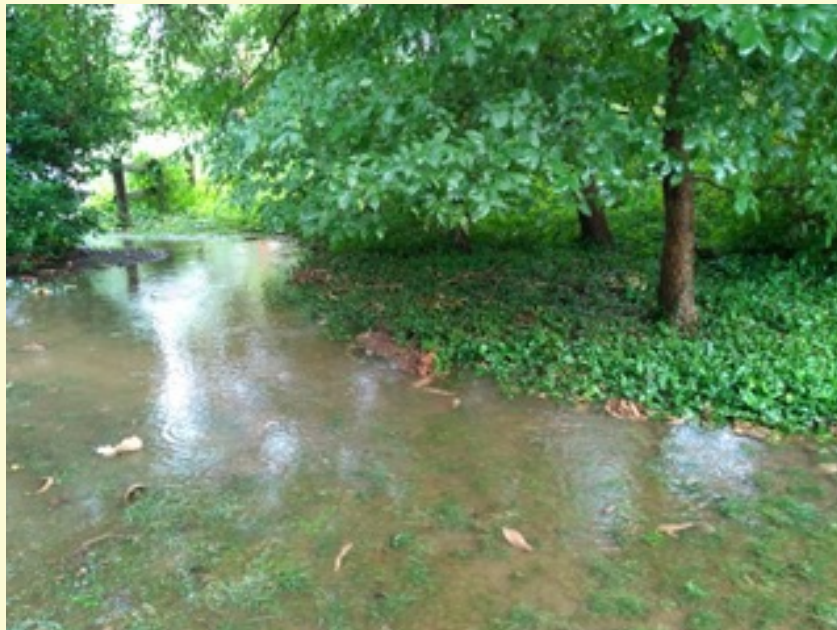
The stormwater problem before the project, flowing south toward Three Oaks (K. Payne photo)
