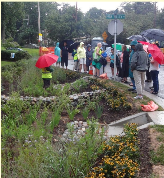
At one of the stormwater projects in the Park Hills neighborhood. (Ed Murtagh photo)
